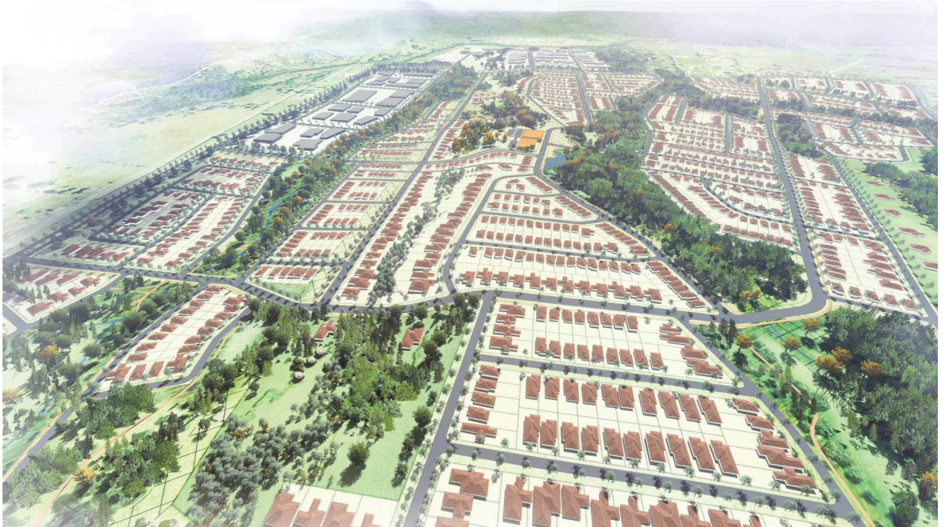
Looking north towards the village centre
